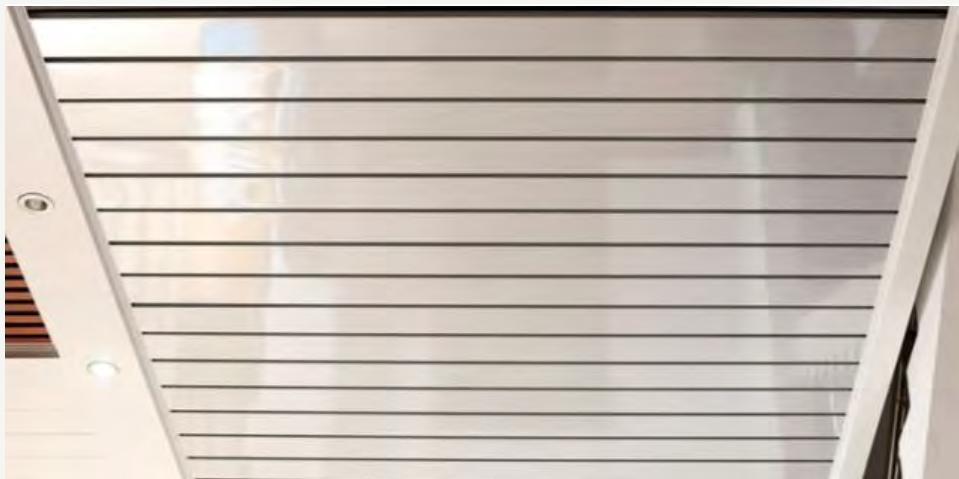
Installed H-profile ceiling
