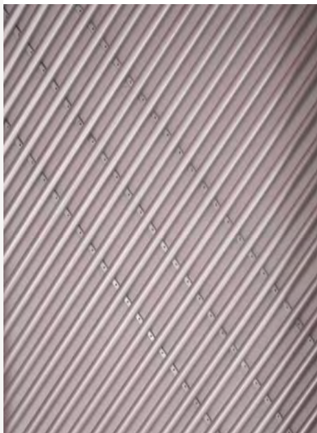
Installed Ø 50 mm tubes
